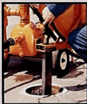
8. Feed hose through guide tube and into storage tank.
