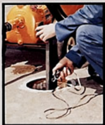
7. Attach ground wire clip to tank.
