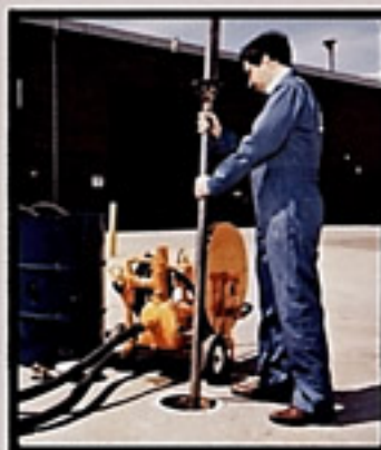
4. Insert guide tube into storage tank.
