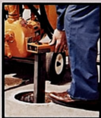
5. Secure hose reel to guide tube.
